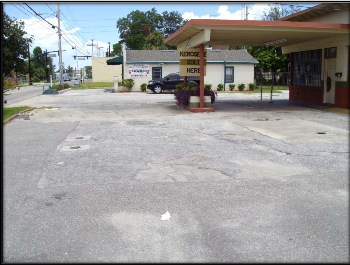
5. View of the front of the vacant business at 927 W. 13 th St. Three apparent monitoring wells are visible.
