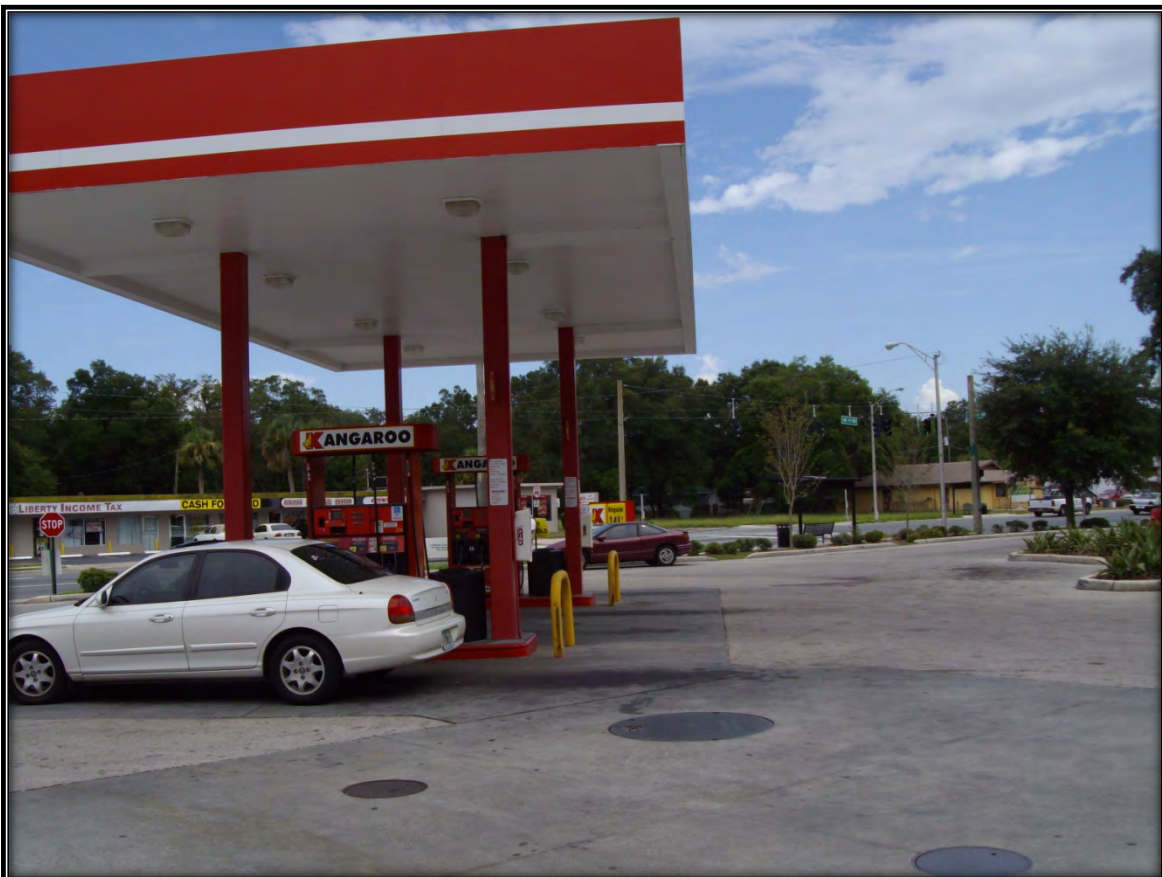
14. View of a gasoline station on the east side of the subject property, facing southeast.
