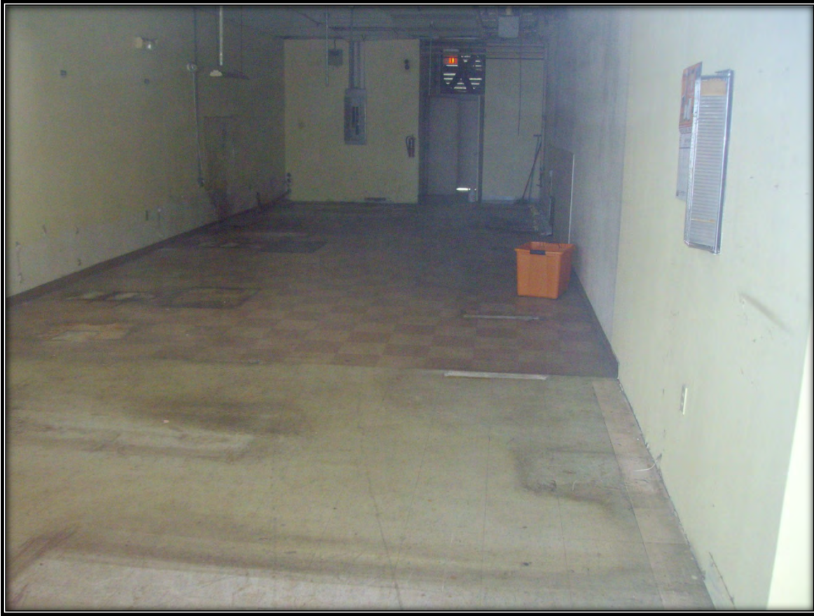
9. View through window of a vacant former dry-cleaning facility on the east side of the subject property.
