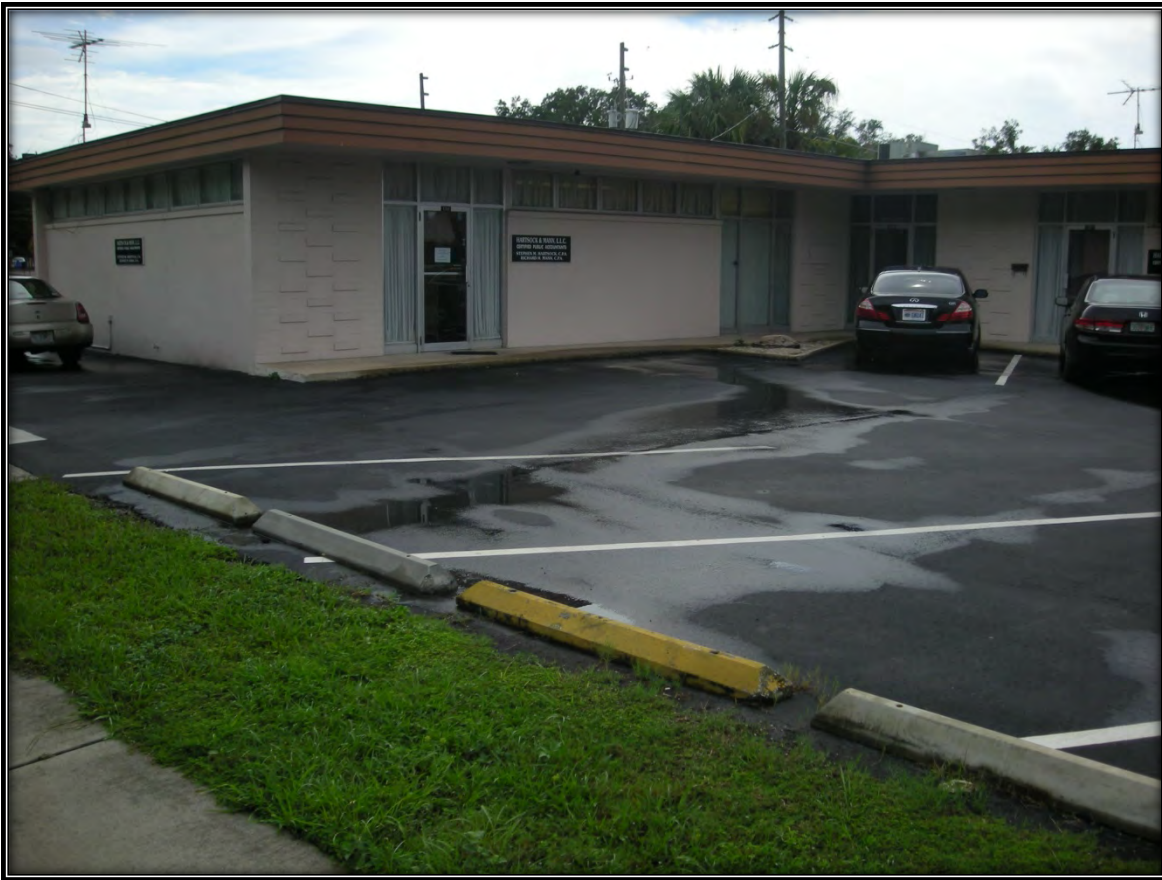
7. View facing southeast from the northeast section of the subject property.
