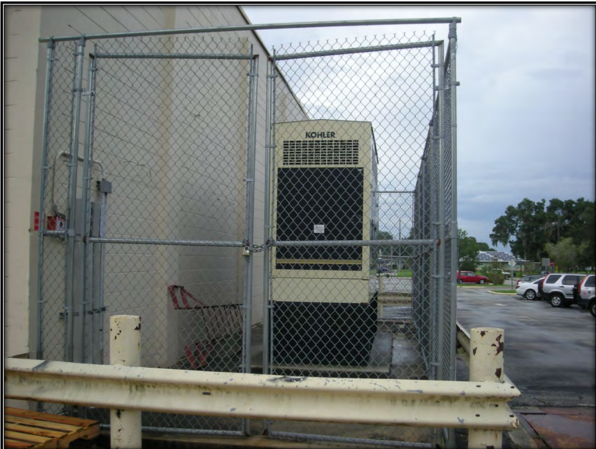
4. View of an approximately 1,000-gallon capacity diesel AST off-site to the north behind a shopping center at 419 E. 1 st Street.
